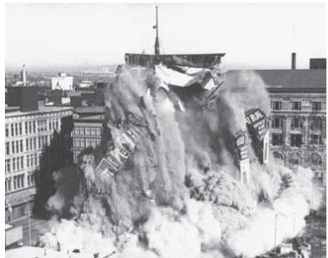
FIGURE 0.7. When the wrecking ball proved too slow, explosives were used, as in this 1970 implosion of the Interstate Trust Building, 1130 Sixteenth Street, an 1891 design by Frank Edbrooke (History Colorado).
