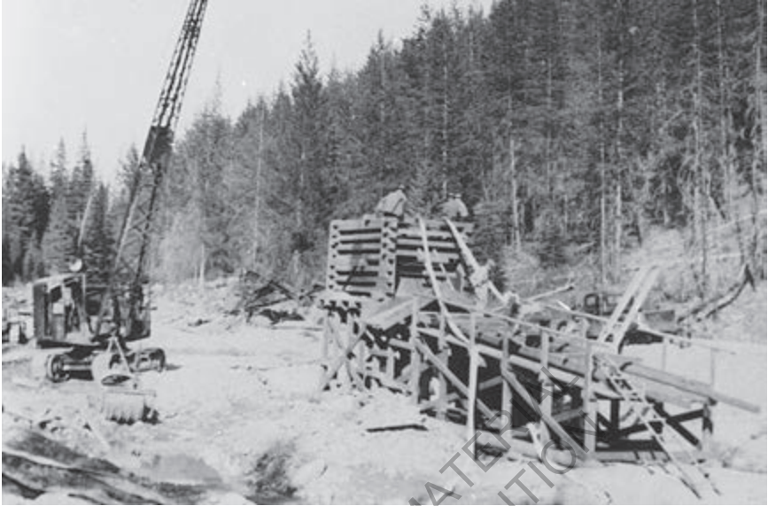
FIGURE 0.2. This dragline dredge was built in 1936 on Red Horse Creek, a tributary of the Red River. Workers are still constructing the washing plant. Courtesy, Idaho Gold Fields Historical Society, Smith Collection, Elk City, ID.
