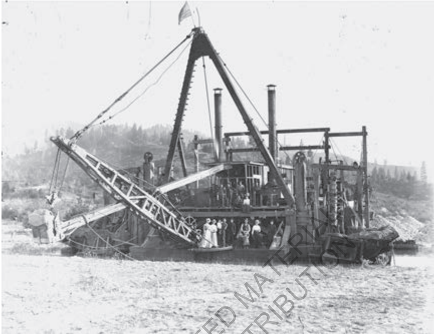
FIGURE 0.1. Like clamshell and orange peel dredges, this ineffective dipper dredge failed to save gold, although it seems to have caught on with the smart set. Courtesy, Idaho State Historical Society, Boise, ISHS 72-112.b.
